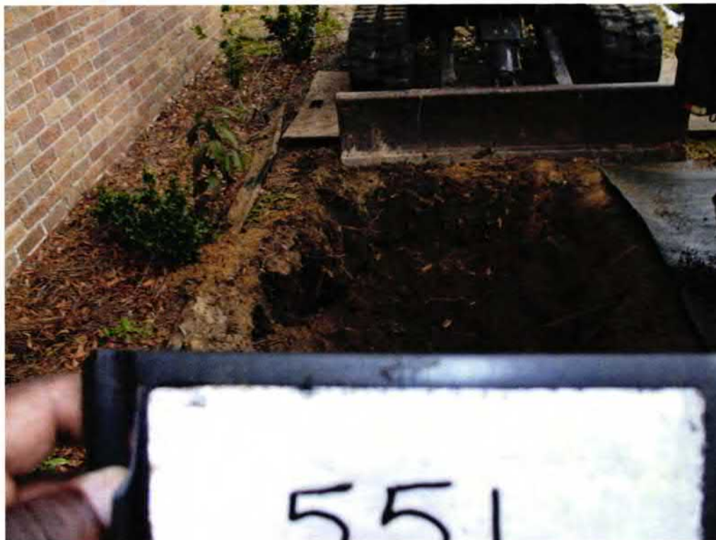
Picture 2: UST 551 Dahlia excavation in progress.
